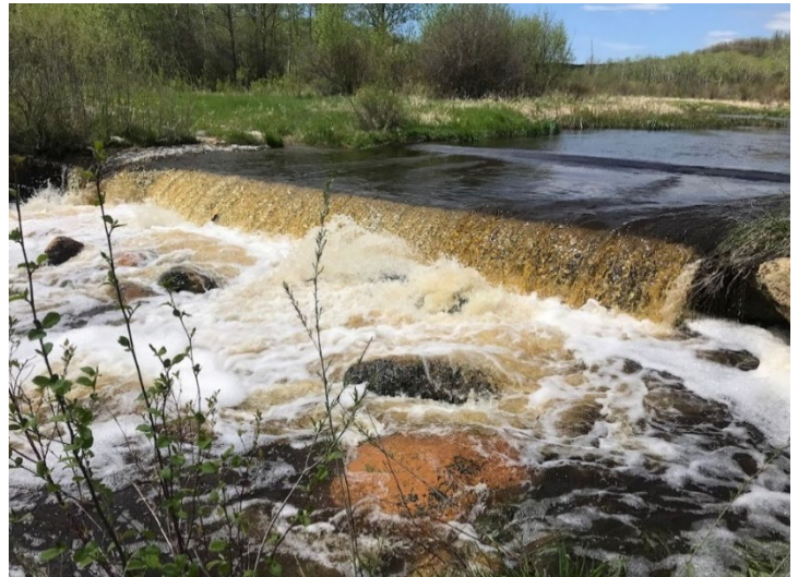
Downstream view of the concrete ford
