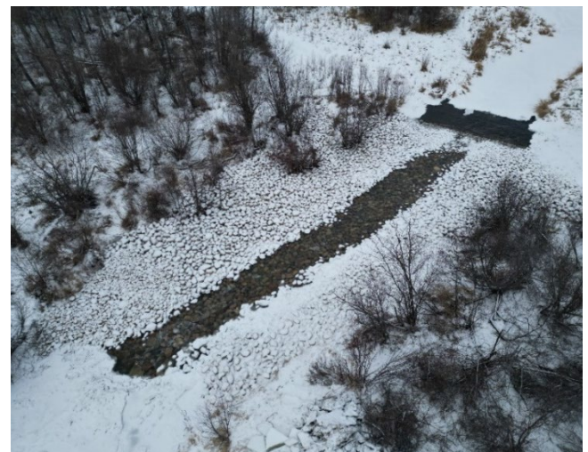
The project site post construction – Dec. 19, 2023
